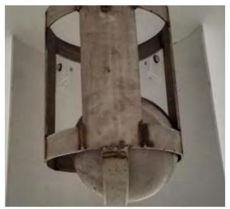
Primary Shutoff Assembly (Collection Tank Interior)
